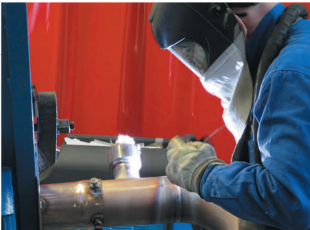
Welding CuNi piping spools
