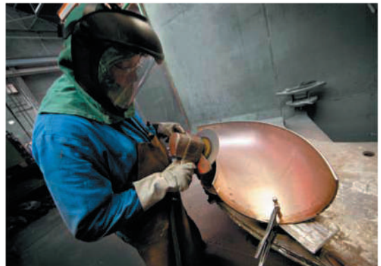
End preparation before welding half shell CuNi elbows
