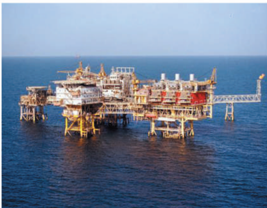
ONGC India, BASSEIN DEVELOPMENT 3 WELL platform "Photography courtesy of LARSEN & TOUBRO, India"
