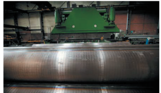
U-BEND PRESS CuNi pipe forming
