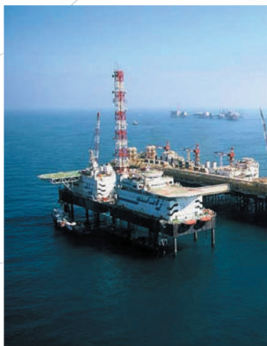
ZADCO UZ750 Oil Field "Photography courtesy of Technip FMC, Emirates"
