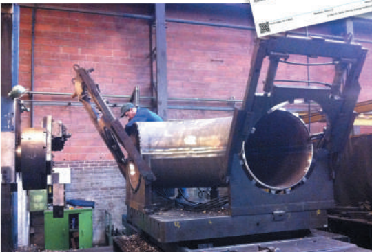
36" CuNi welded elbows
